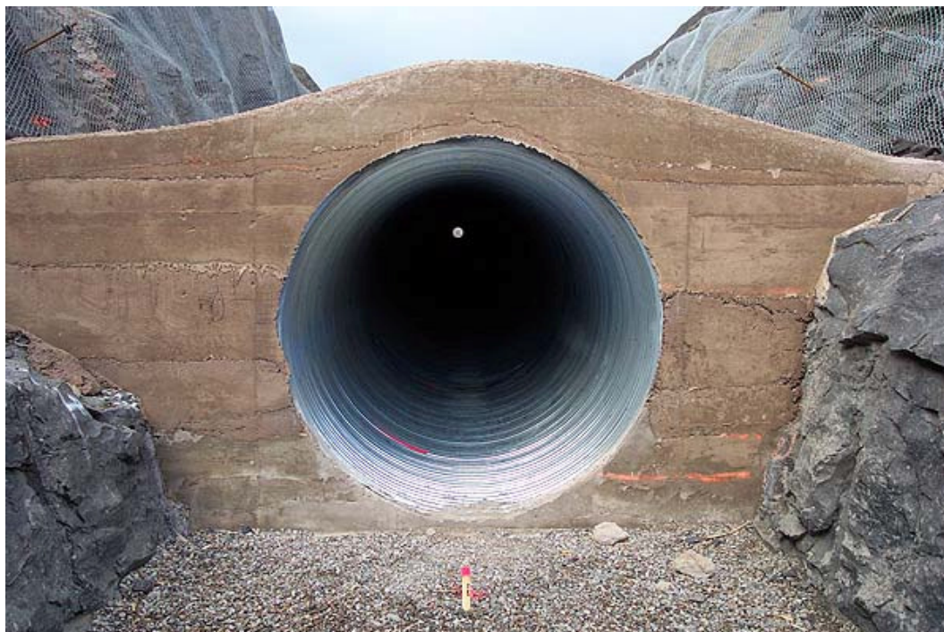
Figure 4 End view showing Flowable Fill Lifts
