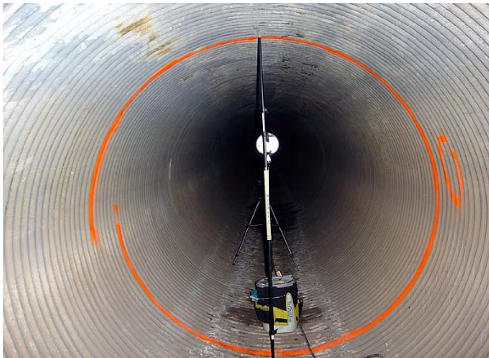
Figure 5 Paint on Corrugation Illustrating Circular Pipe
