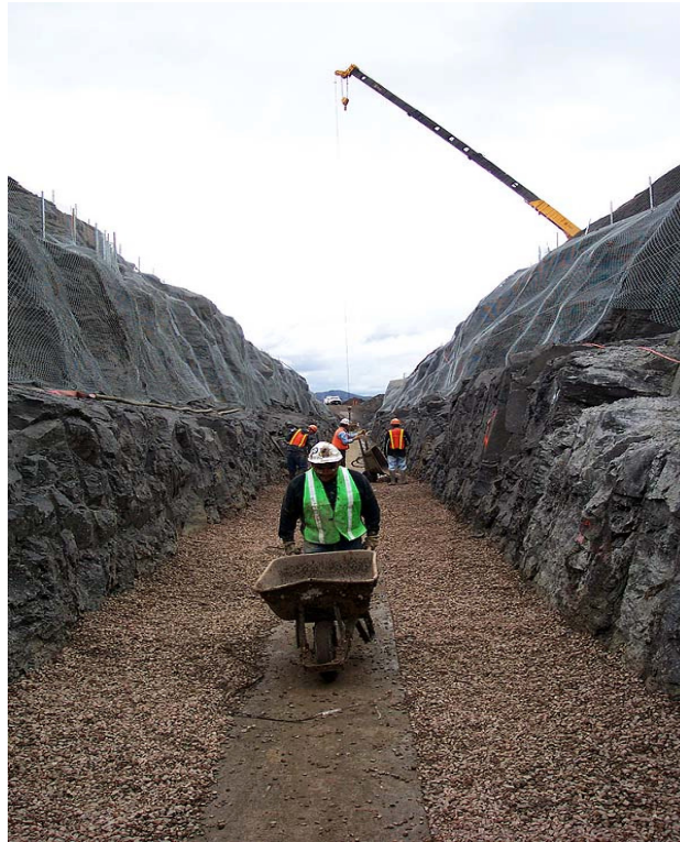
Figure 2 Concrete Strip Foundation for Pipe (note wire mesh protection on trench walls)
