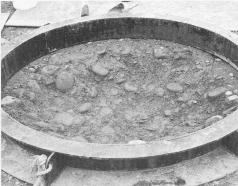
Figure 7. – Test pit during excavation.
