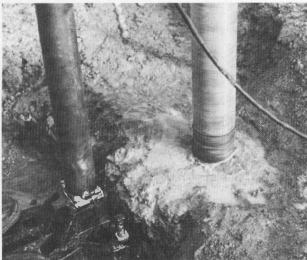
(b) Close-up view of soil-cement coring operation.
